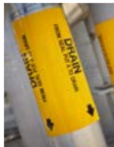
PIPE MARKERS PLACED IN HVAC INSTALLATION
