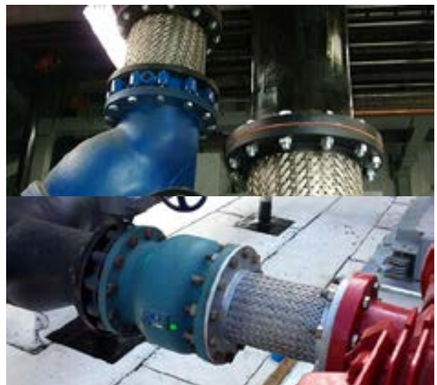
PUMPS WITH FLEXIBLE CONNECTORS IN USE
