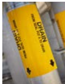
PIPE MARKERS PLACED IN HVAC INSTALLATION
